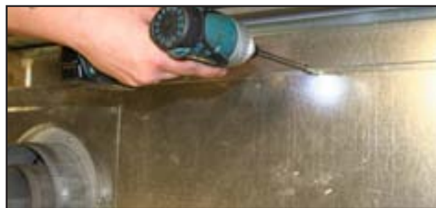
Figure 7. Remove screws from top of the unit
