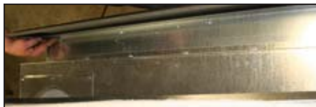
Figure 7a. Remove shell from the top of unit. Remove screws from outer edge.
