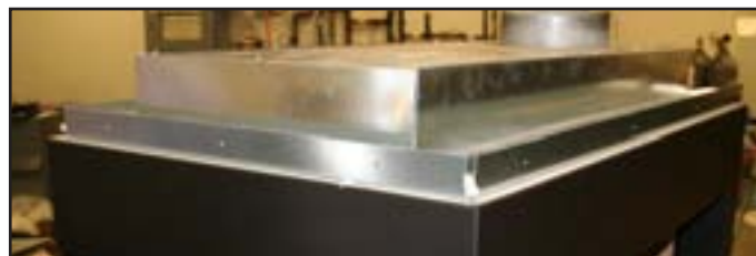
Figure 7c. Finished removing Nailing Flange extension.
