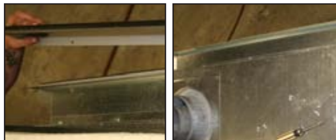
Figure 7b. Remove the nailing flange extension from the unit. Reinstall shell. Screw shell in place.
