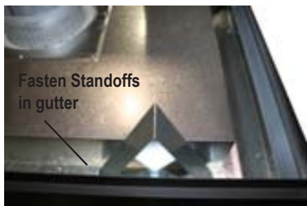
Figure 6. Installing the H*38PR* standoffs.
