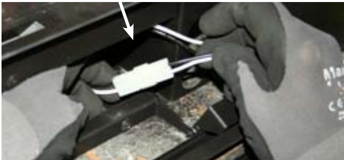
Figure 10b. Connect Fan Speed Control wires.
