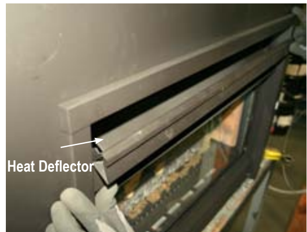
Figure 9b. Installing the upper louvres.
