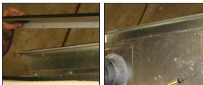
Figure 7b. Remove the nailing flange extension from the unit. Reinstall shell and insulation. Screw shell in place.
