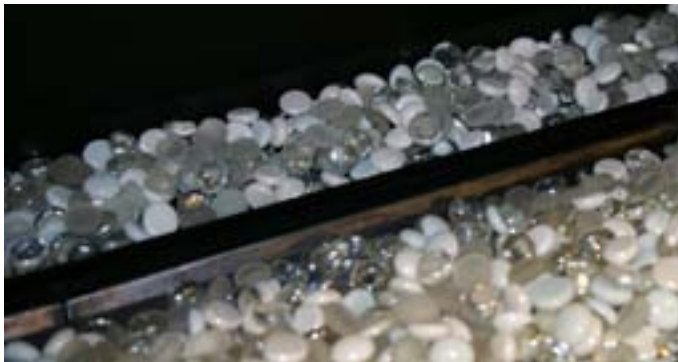
Figure 26. Completed firestone installation. (Note: DO NOT place ANY firestones on top of the burners or pilot).
