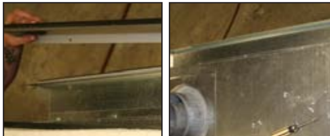
Figure 7b. Remove the nailing flange extension from the unit. Reinstall shell and insulation. Screw shell in place.
