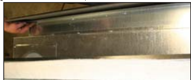
Figure 7a. Remove shell and insulation from the top of unit. Remove screws from outer edge.
