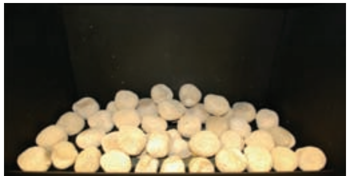
Figure 32s. Completed faux Rock installation.
