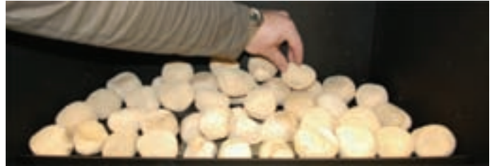
Figure 32p. Place the sixth Top faux Rock on top, behind the pilot burner faux Rocks.
