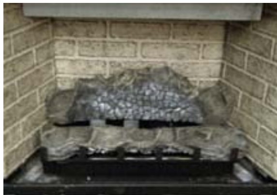
Figure 29c. Front Log placement.
